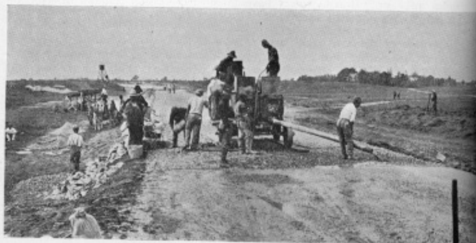
LONG ISLAND PARKWAY CONSTRUCTION—THE FINISHING MACHINE
