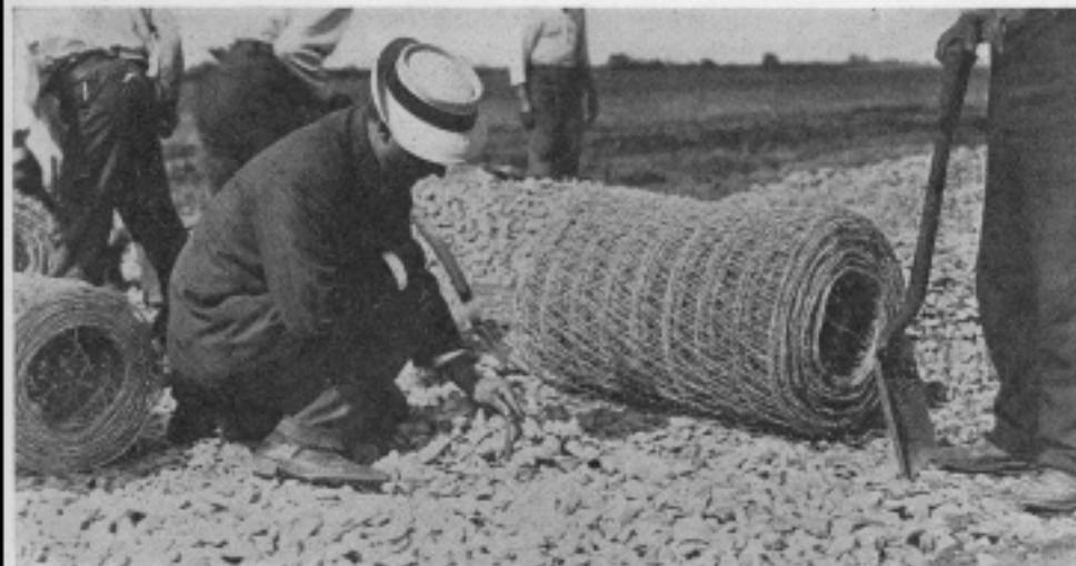
CONSTRUCTING THE CEMENT PARKWAY
